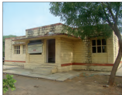
Fig. 4. The project was implemented in vacant staff quarters behind the community health centre in Gulbarga, Karnataka.
